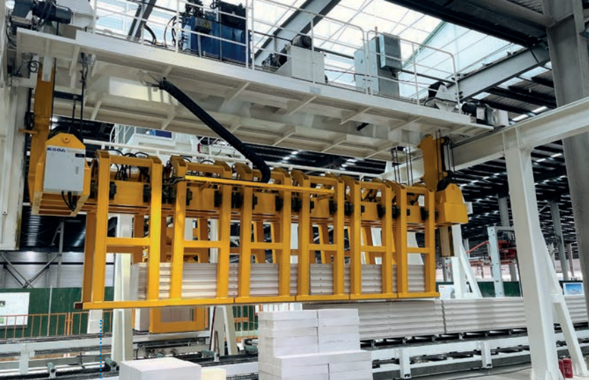
Panel sorting crane in the HGA Anhui plant.
