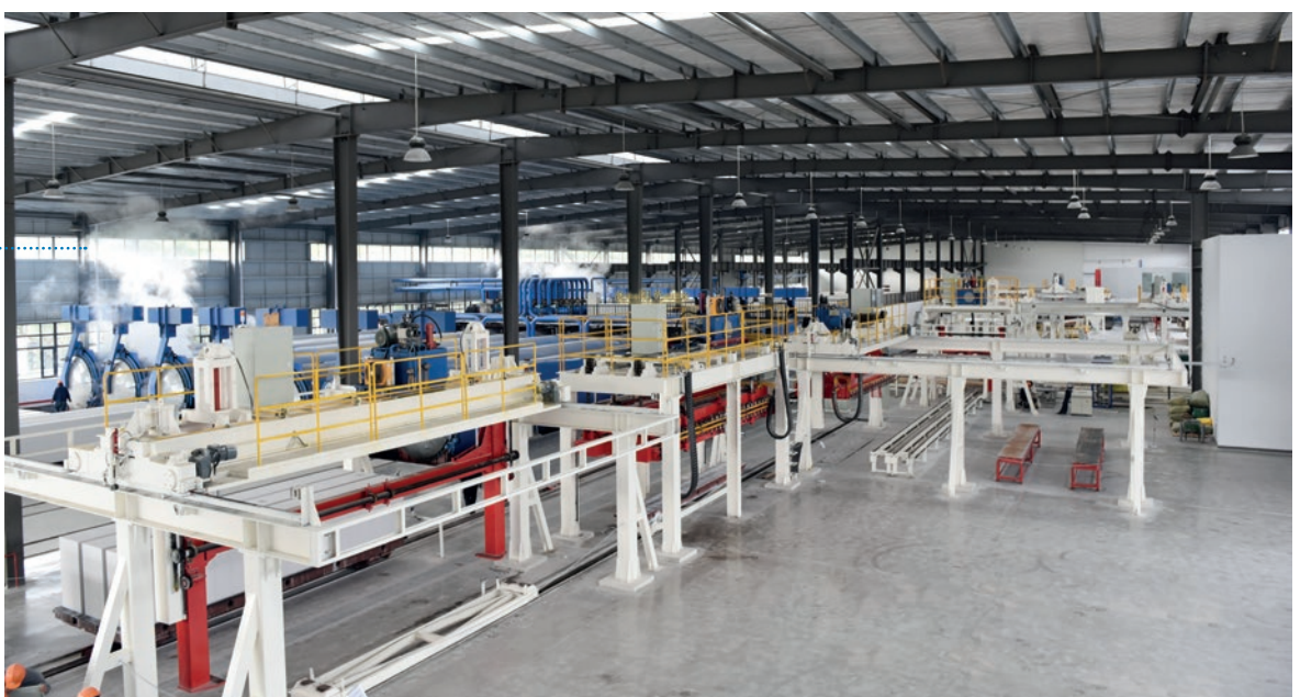
General overview of the plant.
